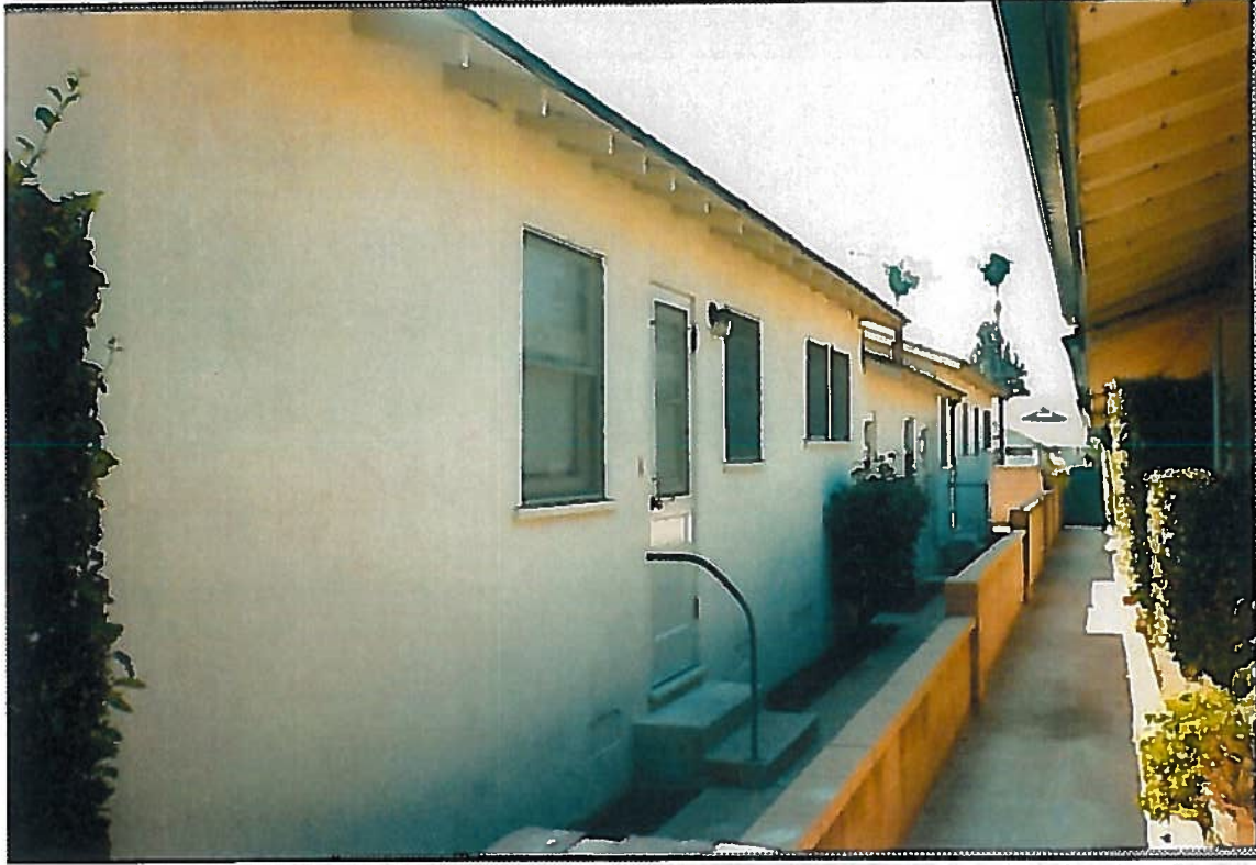
REAR VIEW OF SUBJECT
