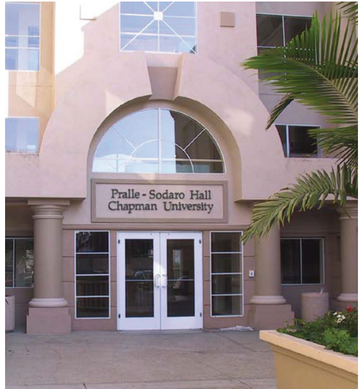
Building Identification/Wall Sign Example
