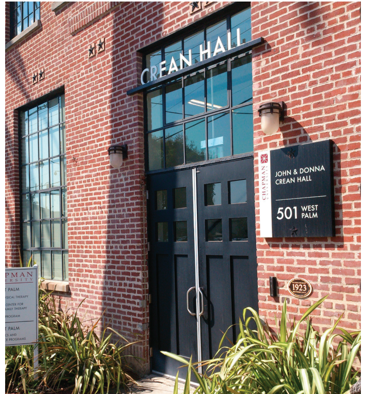
Building Address/Entry Wall Sign
