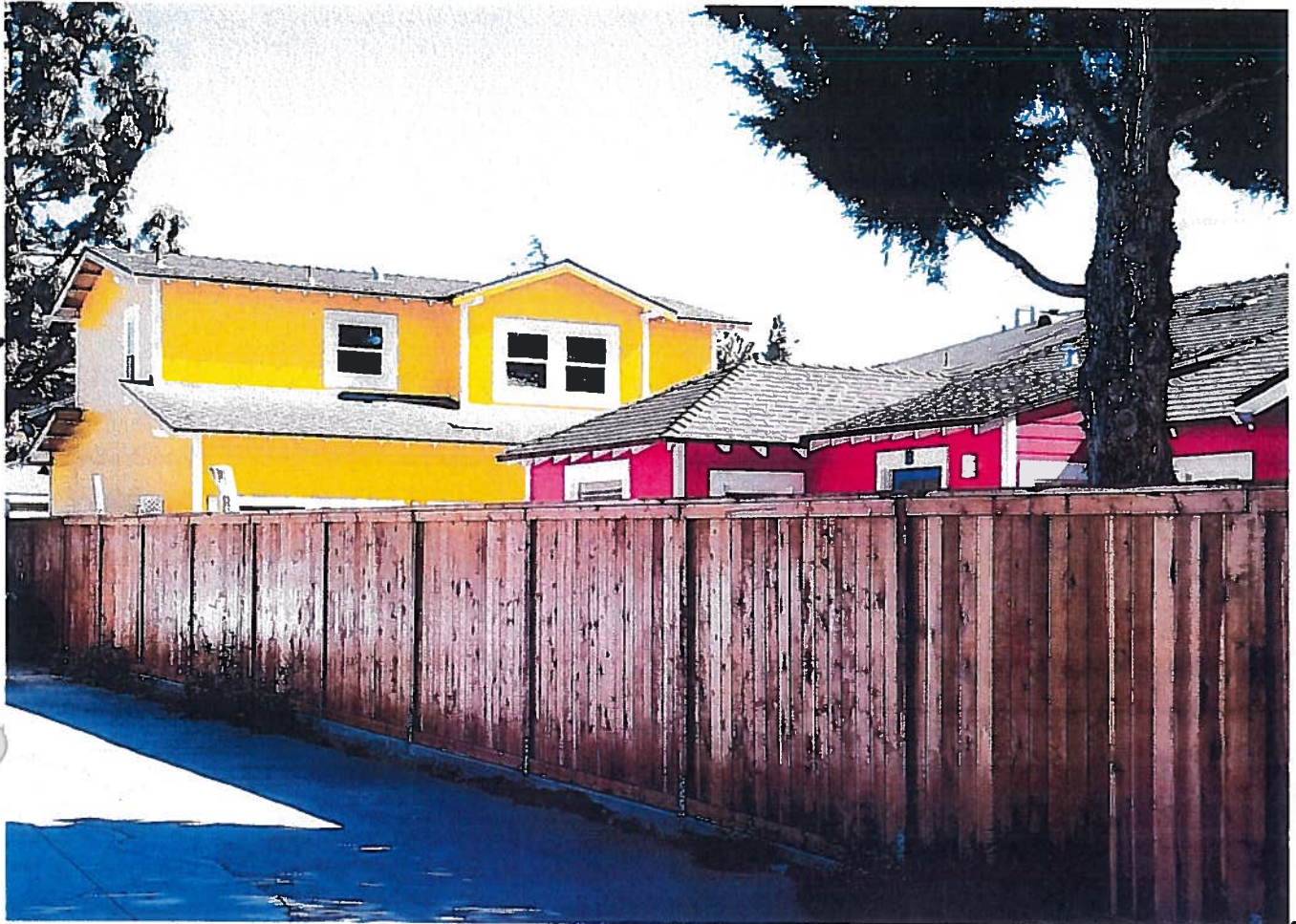
Note: Rear House Pediment made to look exactly with the old front
