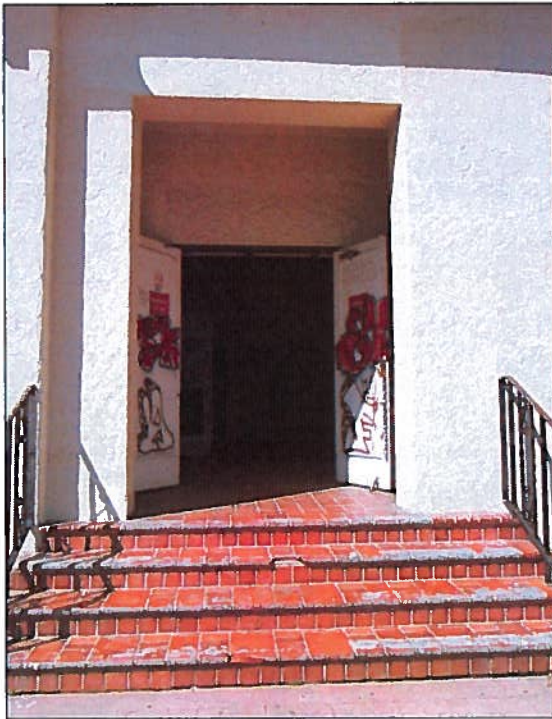
Figure 17: Secondary Entrance. Secondary entrance in east elevation (March 17, 2016).
