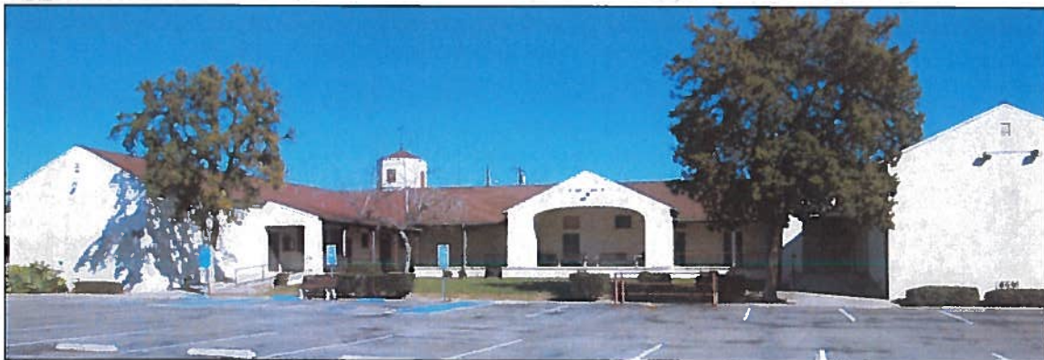
Figure 3: West Elevation. View to the east (February 9, 2016).
