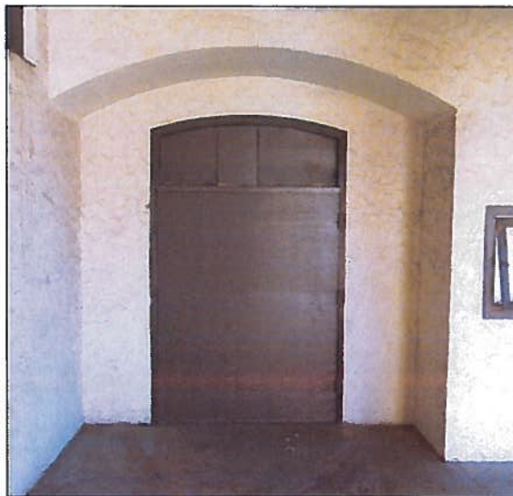
Figure 9: Alcove Detail. Detail of arched alcove and door with segmental arched transom in west elevation (February 9, 2016).
