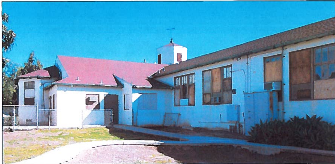
Figure 6: North Elevation. View to the east. Note bay window on left side of photograph.
