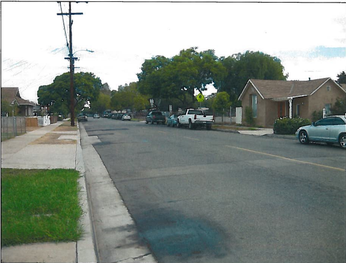
4. N. Lemon Street at intersection with W. Walnut Avenue. View northeast.
