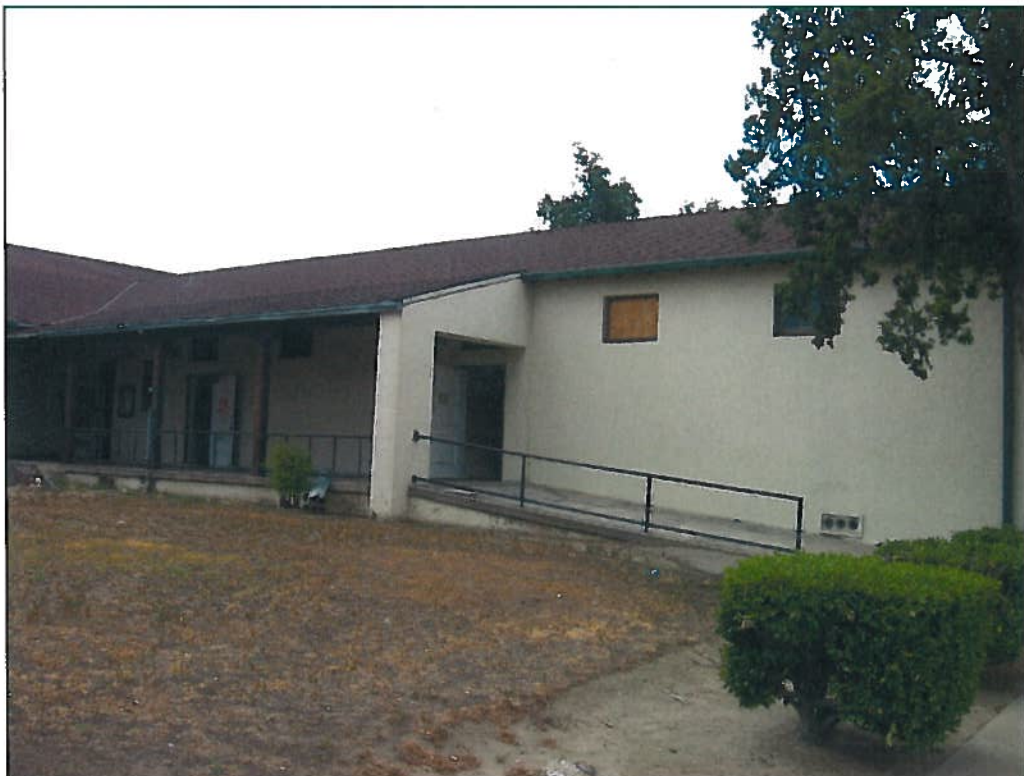
South building wing from courtyard. View southeast.
