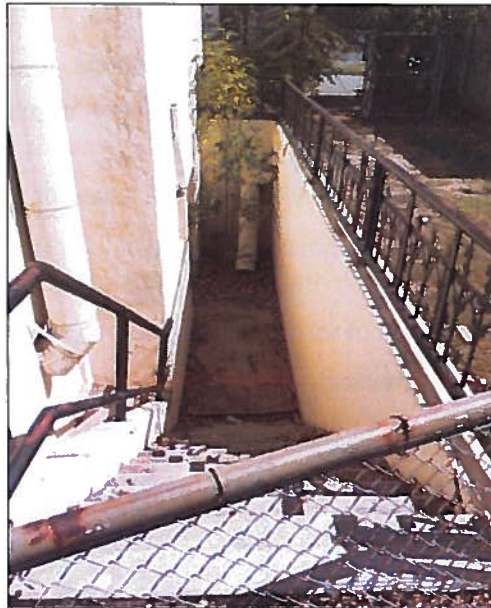
Figure 25: Basement Steps. Basement steps and wrought iron railing at south end of the building (October 3, 2015).
