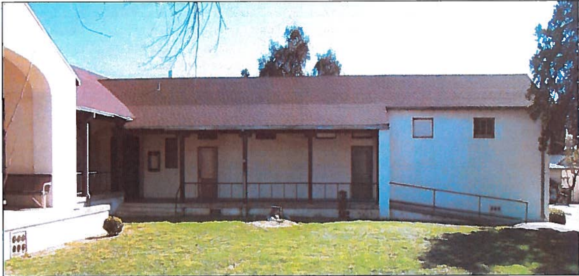
Figure 5: South Wing of West Side. View to the south (February 9, 2016).
