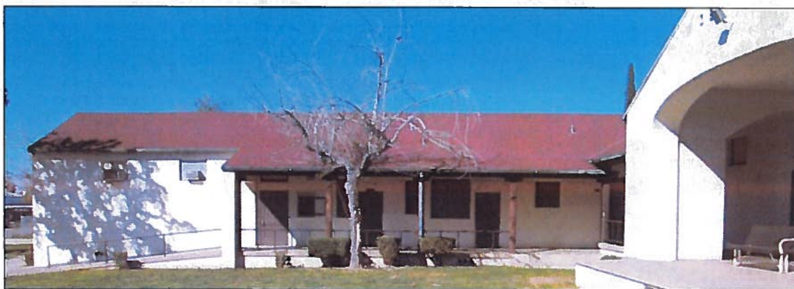
Figure 4: North Wing of West Side. View to the north (February 9, 2016).
