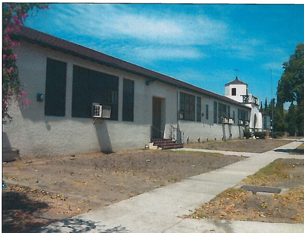
East elevation on N. Olive Street. View northwest.
