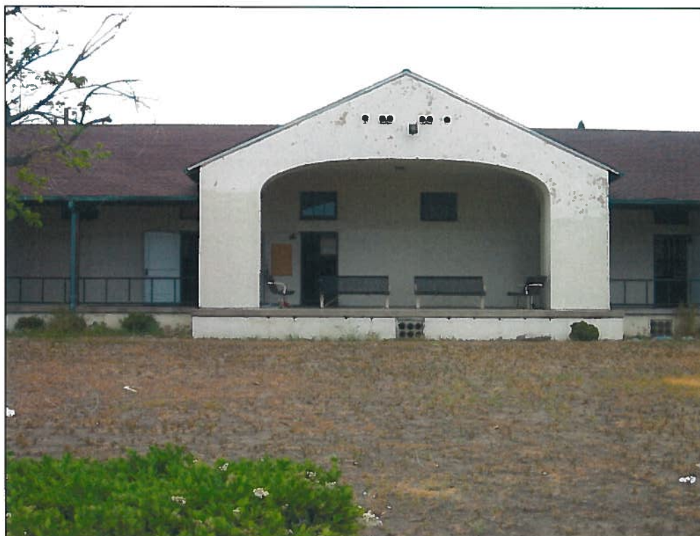
Courtyard and stage. View east.
