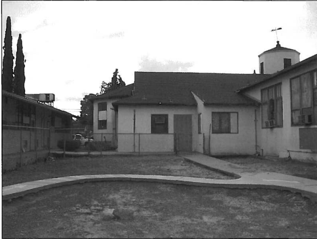
Tower element and projecting bay on north side of building. View east.
