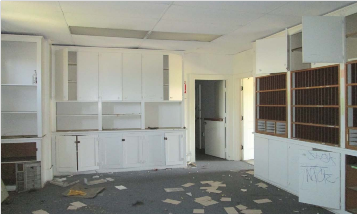
Figure 21: Administration Room. Administration room with built-in cabinets and shelves (March 18, 2016).
