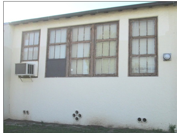
Figure 18: East Elevation Detail. Detail of east elevation wood-framed windows, canale vents, and eave (February 9, 2016).
