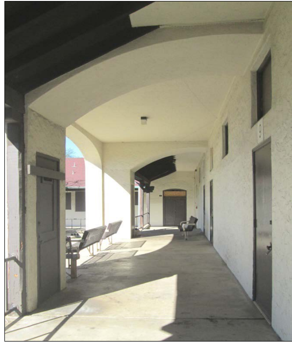
Figure 8: Walkway Detail. Detail of arcaded walkway, view to the north (February 9, 2016). Note clerestory windows.
