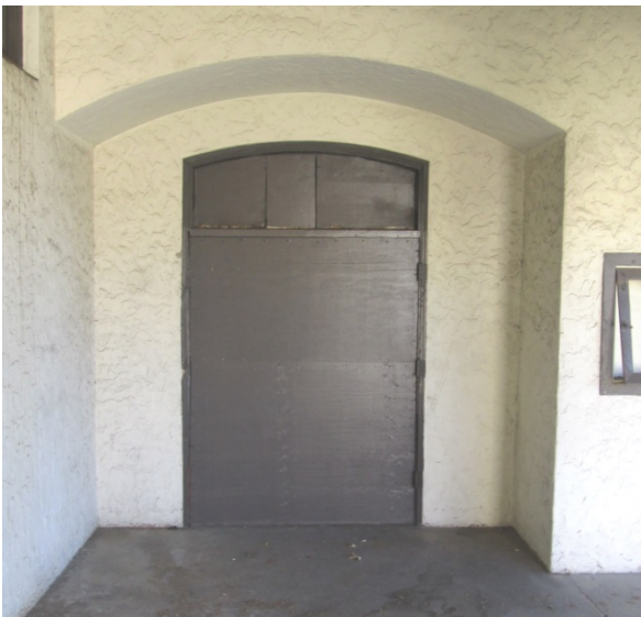
Figure 9: Alcove Detail. Detail of arched alcove and door with segmental arched transom in west elevation (February 9, 2016).
