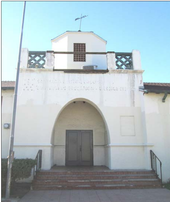
Figure 15: Primary Entrance. Primary entrance and tower, view to the west (February 9, 2016).
