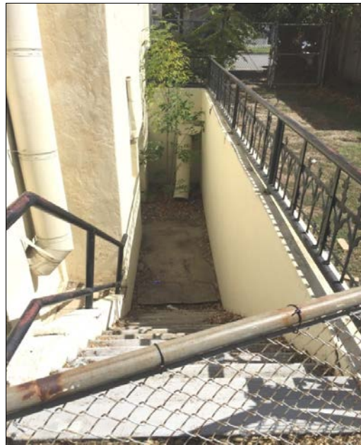
Figure 25: Basement Steps. Basement steps and wrought iron railing at south end of the building (October 3, 2015).
