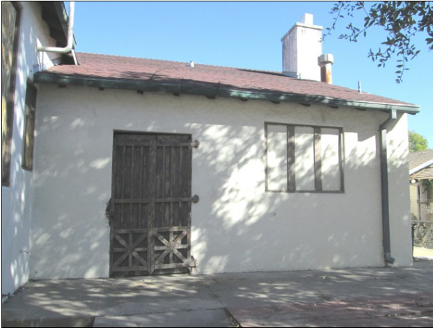
Figure 11: West Elevation View to the East. Southern portion of west elevation, view to the east. Note the chimney (February 9, 2016).
