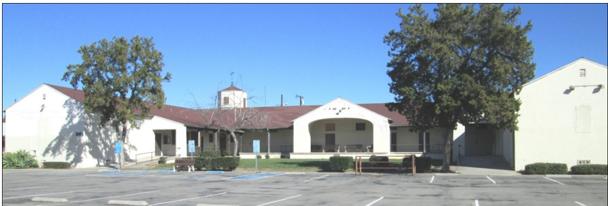
Figure 3: West Elevation. West elevation, view to the east (February 9, 2016).
