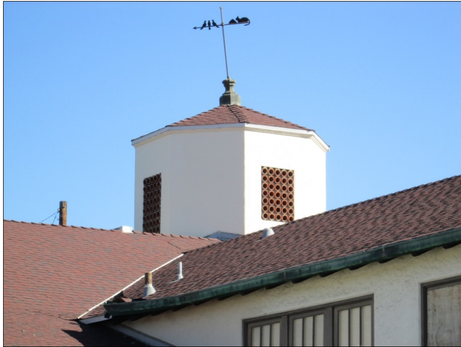
Figure 19: Northeast Tower View. Tower, view to the northeast (February 9, 2016).
