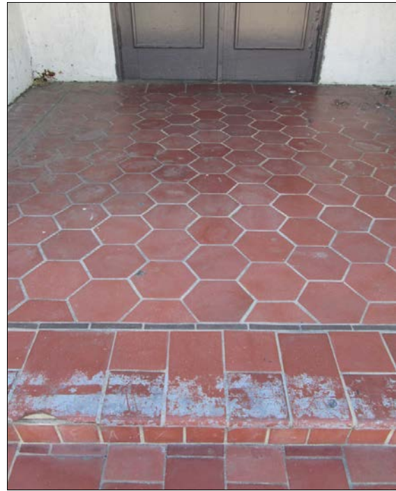
Figure 16: Tile Detail at Entrance. Detail of terra cotta tile at the primary entrance (February 9, 2016).
