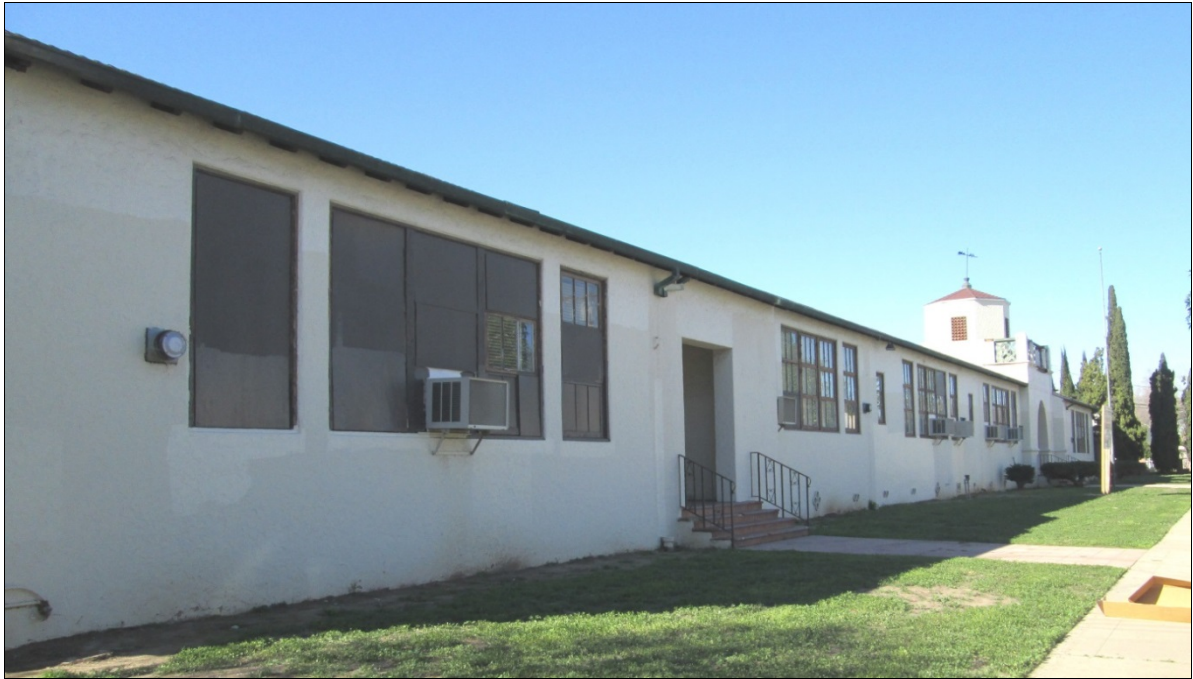
Figure 14: East Elevation View to Northwest. East elevation, view to the northwest (February 9, 2016).
