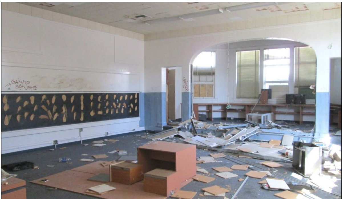
Figure 20: Auditorium and Bay Window. Auditorium with stage and bay window at northeast end of main building (March 18, 2016).
