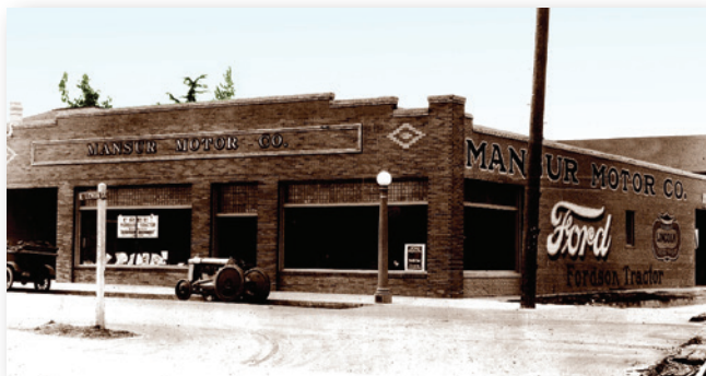
Now home of Snooze AM Eatery, here's the building at 240 W. Chapman when it opened as a Ford dealership in 1922.
