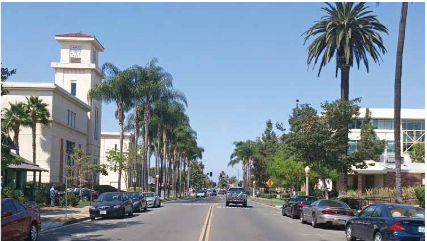
Kennedy Hall and Beckman Hall Looking North on Glassell Street
