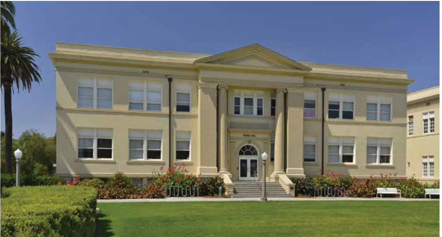
Reeves Hall (formerly the Education/Art Building) - opened 1913
